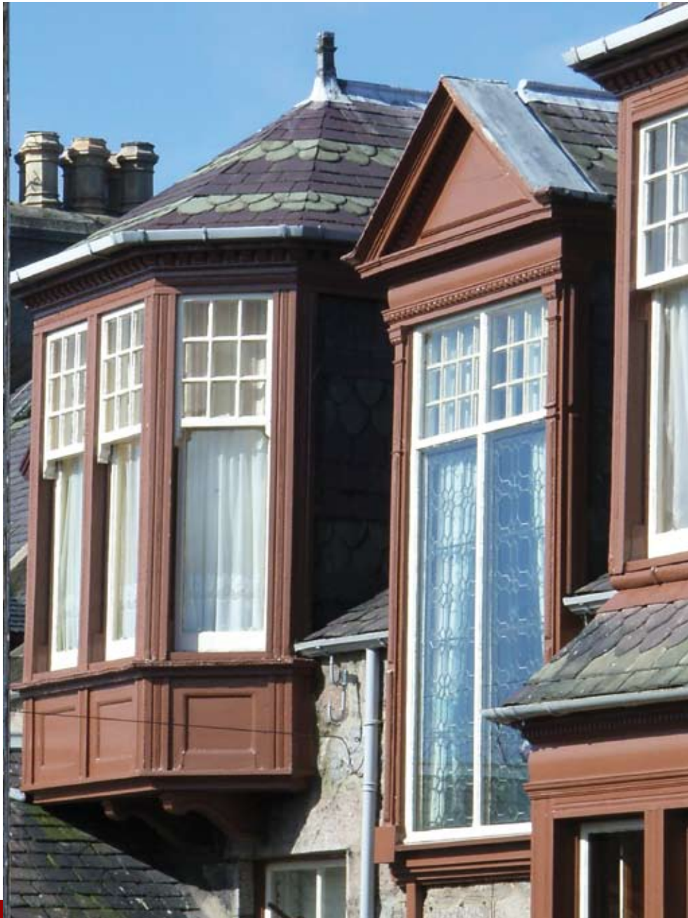
Traditional joinery detailing, West End
